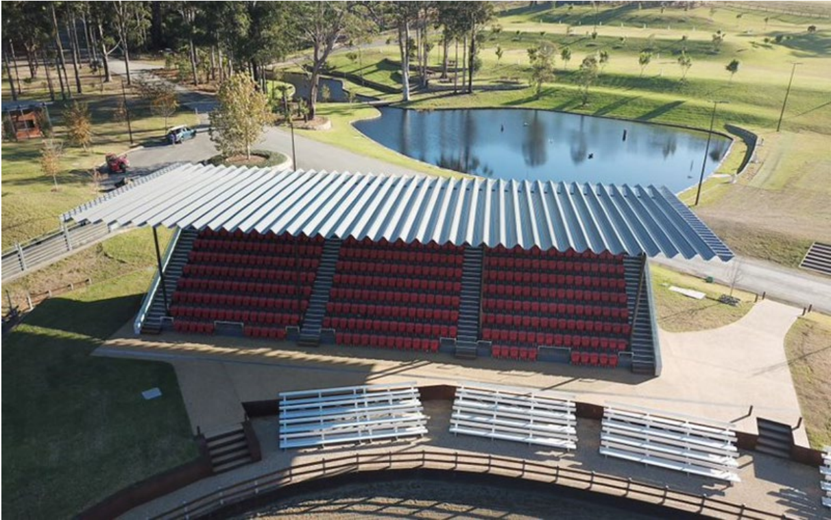
ARAMAX wide span roofing is rolled on site. Image courtesy Bay & Coast Metal Roofing.
